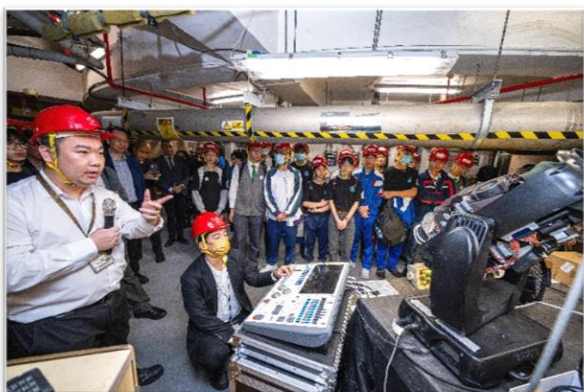
GEG offered students a close-up look at the operation system of various performance installations to expand technological horizons.
